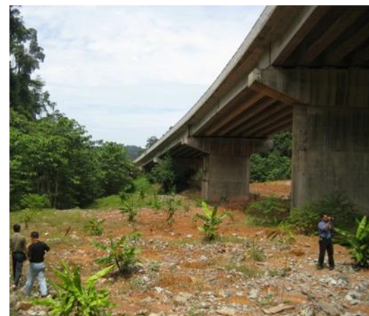
Figure 4.2: Existing viaducts along the Gua Musang – Kuala Berang Road
